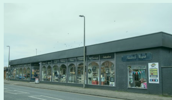
This modern building has been made more respectful of its historic environment by breaking up the wide expanse of window with mullions.
