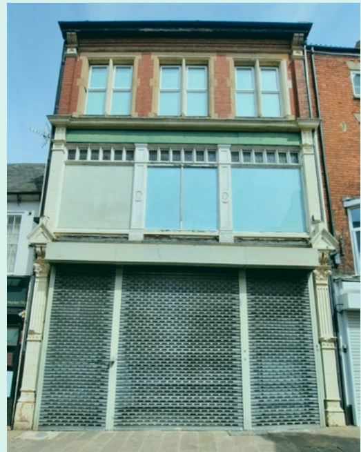
Removable grilles allow customers to see shop displays even when the business is closed. Permanent fixing points are discrete and do not detract from the shopfront.
